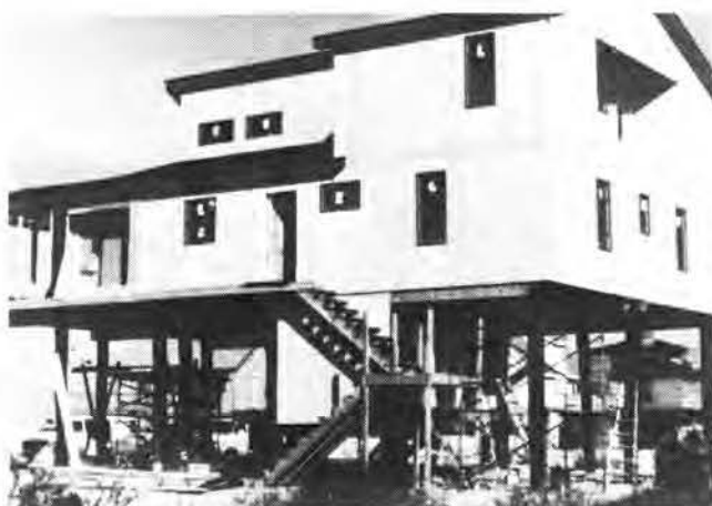
Figure 4.14. Pile Foundations
