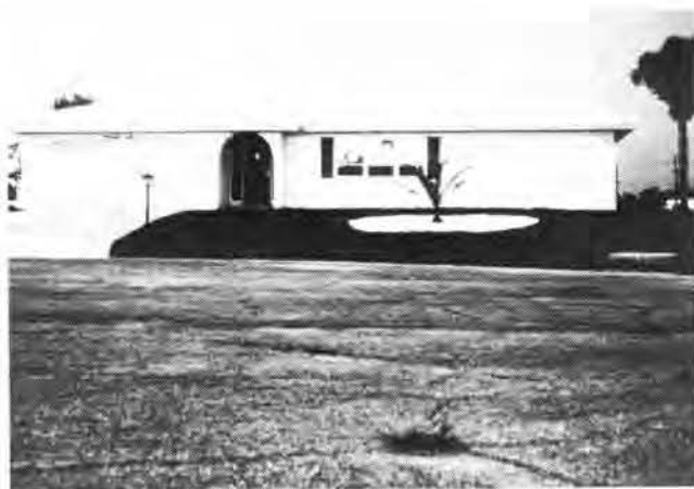
Figure 4.1. Elevation by Earth Fill
