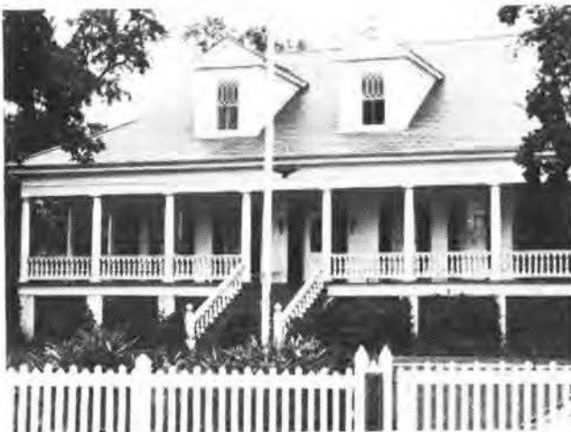
Figure 4.15. Pier Foundations
