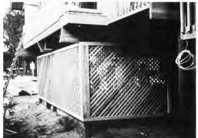
Figure 4.54. Breakaway Walls
