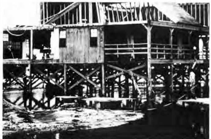
Figure 4.23. Diagonal Bracing
